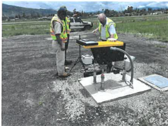
Installation of the PAPI LED Lights
