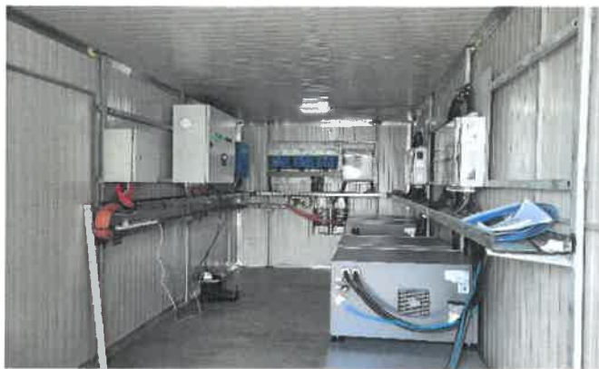
Containerised Hybrid 48 Volt Solar system
